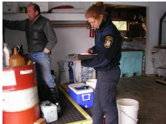
Diesel fuel protected with 110% containment
