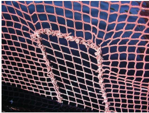
Net repair completed on the jump net portion of a containment net
