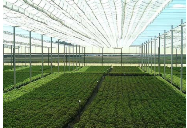
Figure 17. Retractable roof greenhouses are very versatile; automation enables variable shade control and excellent ventilation.
