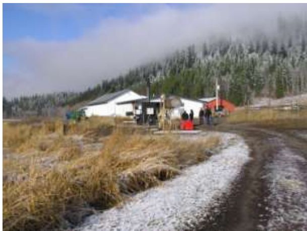
Riverside Meats Inciner8 incinerator with diesel tank
