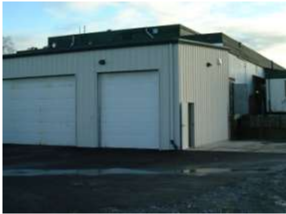
Pitt Meadows Meats New waste handling building
