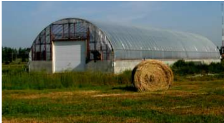
Kawano Farm Non-SRM Composting Structure
