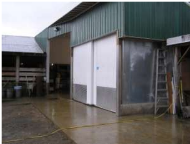
Gunter Bros. Meat Co. Cold Storage Building
