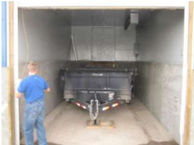
Country Locker New Refrigeration Room and Waste Trailer
