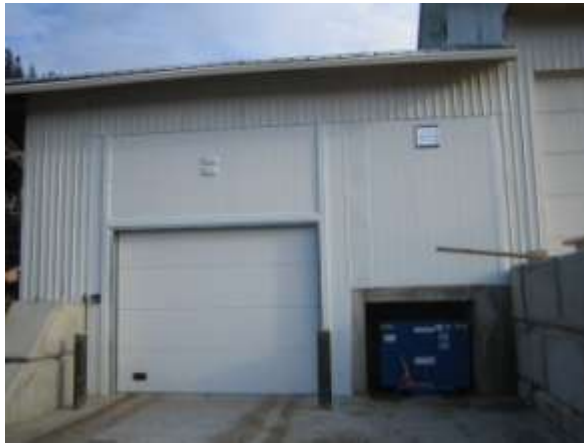
Rodear Meats Refrigerated Waste Storage Room.
