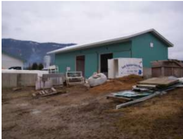
North Okanagan Game Meats Cold Storage and Potential Incinerator Housing
