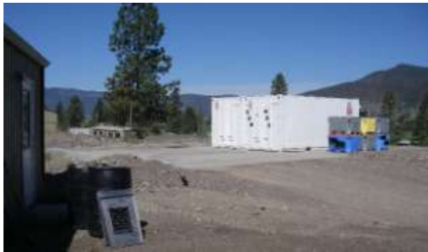
Medallion Meats SRM Storage Containers on Concrete Containment Slab
