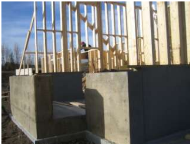
Northwest Premium Meat Cooperative Waste Storage Room Construction Underway
